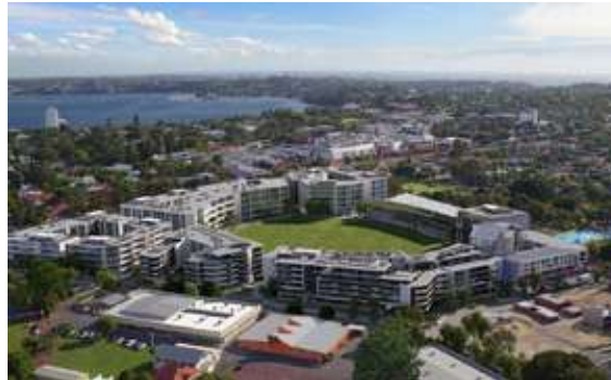
Figure 1 - Claremont on the Park (Source: LandCorp)
